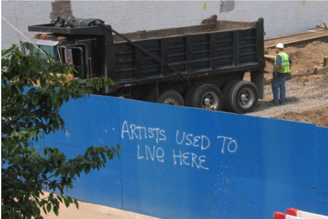
Still from Gut Renovation, 2012, 81 minutes.
